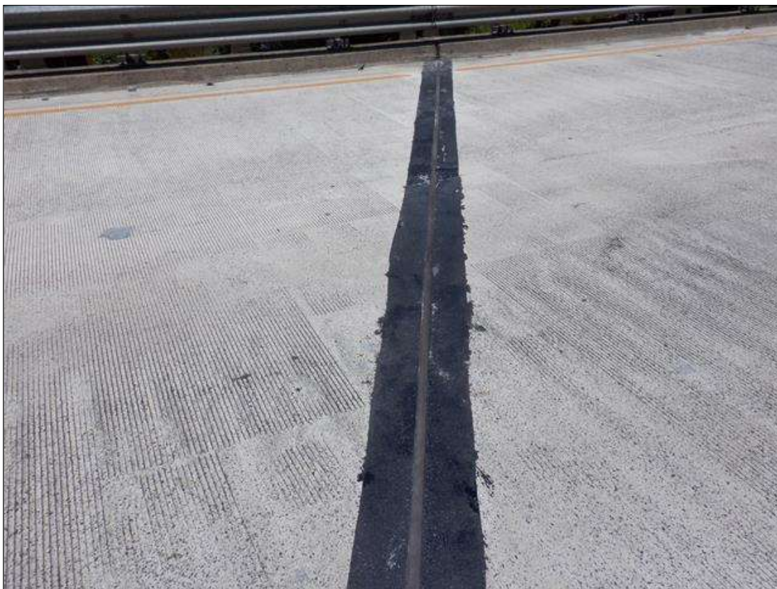
BENT 8 EXPANSION JOINT
