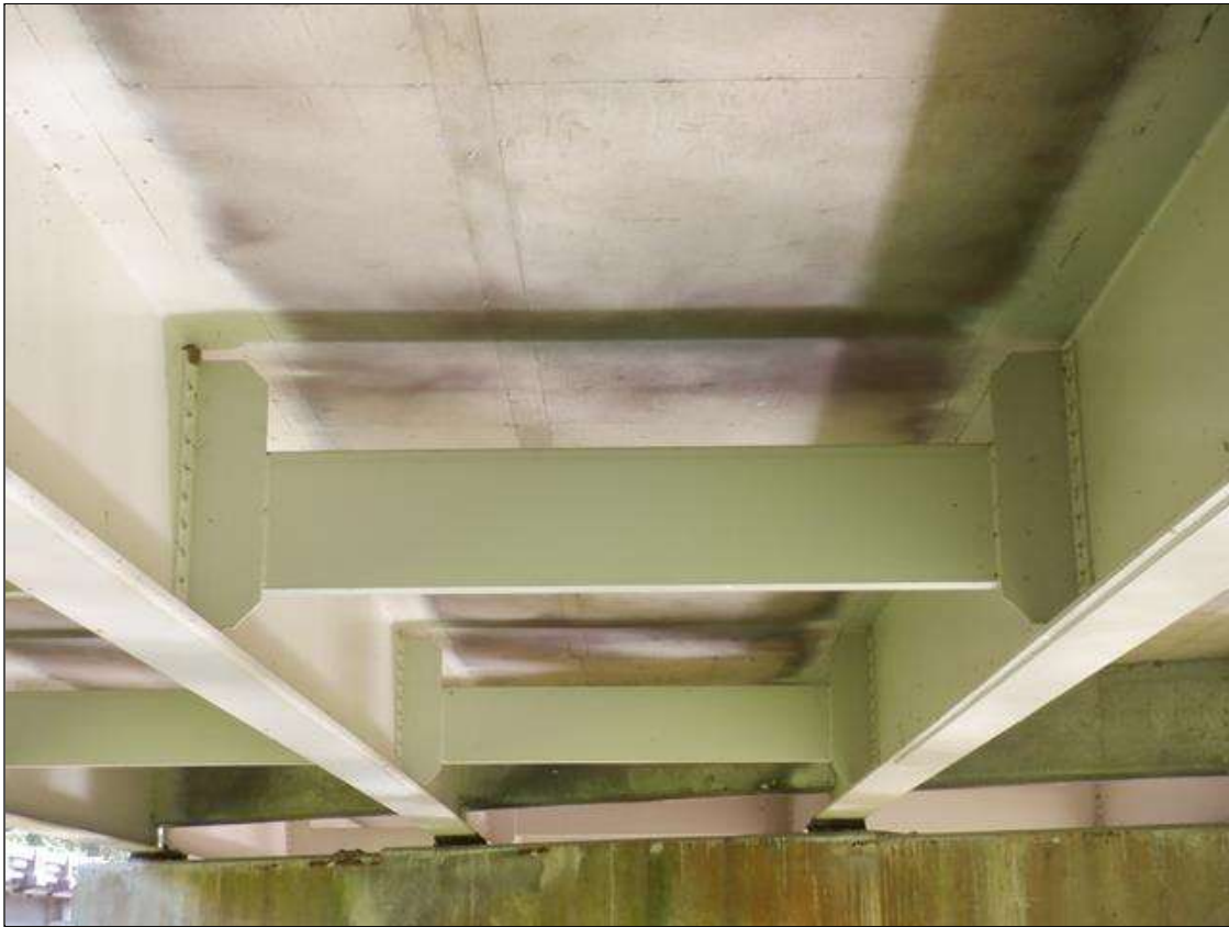
SPAN 3 BAY 2 INTERMEDIATE DIAPHRAGM
