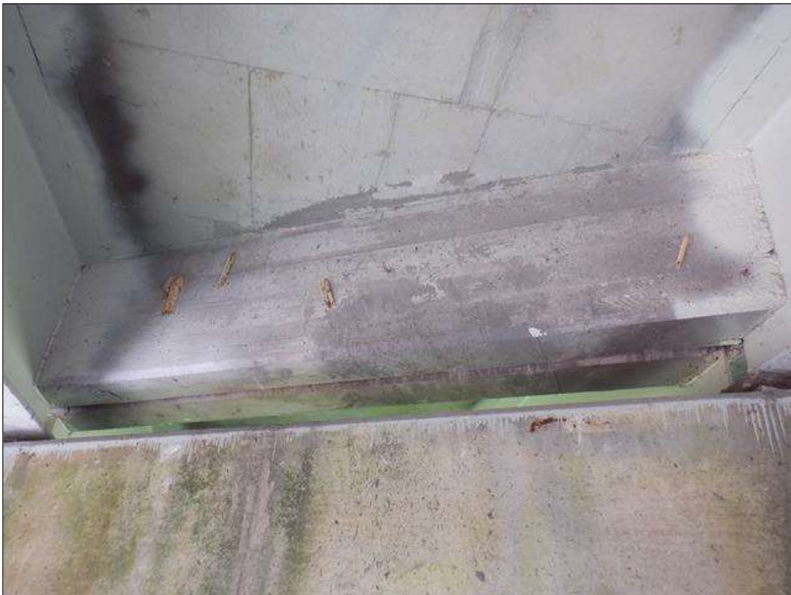
SPAN 3 BAY 2 NEAR DIAPHRAGM
