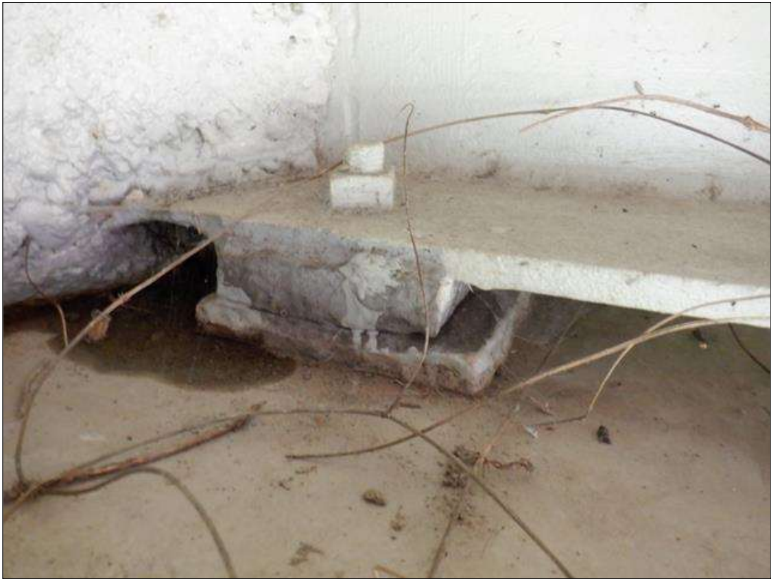
SPAN 1 BEAM 3 NEAR BEARING
