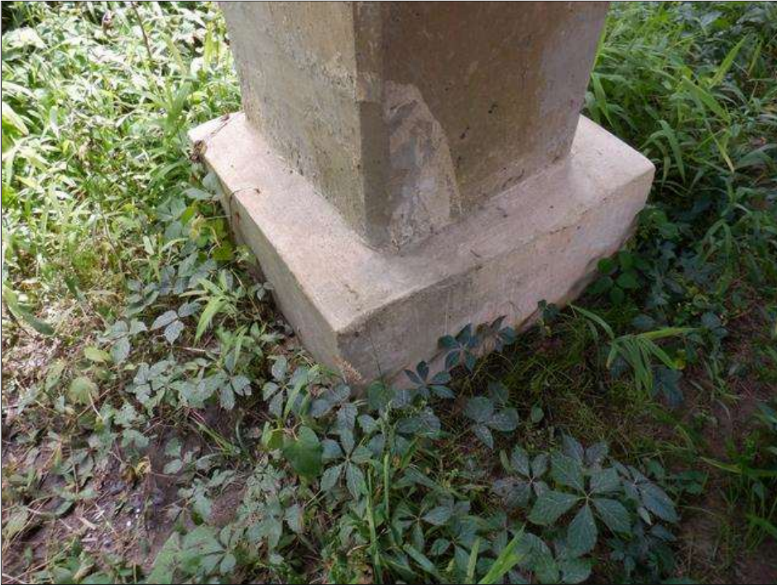
Bent 7 Pile 7: 15 INCHES WIDE X 10 INCHES HIGH AREA OF THE SOUTH FLANGE EXHIBITS HEAVY SURFACE CORROSION WITH SECTION LOSS ON WEB AND FLANGES OF EXPOSED STEEL PILE AT GROUNDLINE. UP TO 0.50 INCH SECTION REMAINING. NORTH FLANGE AND THE WEB EXHIBIT HEAVY SURFACE CORROSION WITH NO MEASUREABLE SECTION LOSS. CONCRETE REPAIR AT BASE OF PILE COVERS STEEL PILE.
