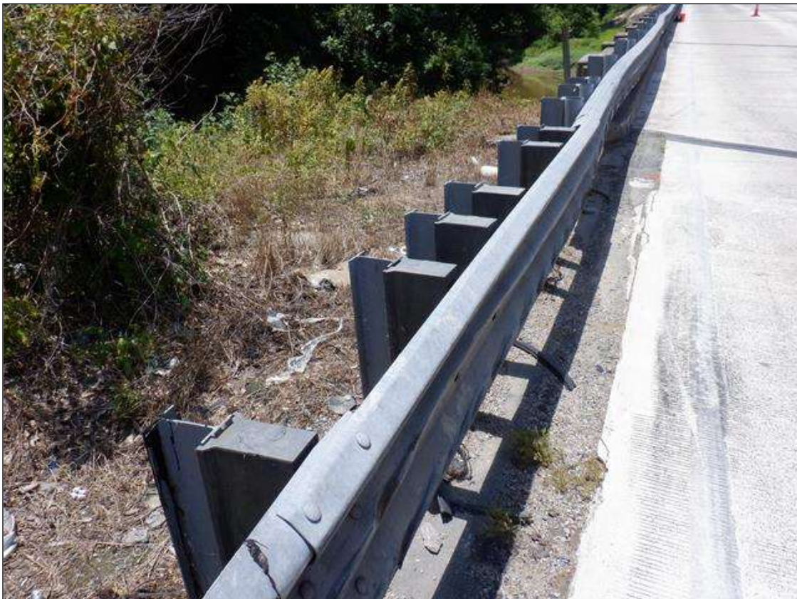
NORTHEAST GUARDRAIL TRANSITION
