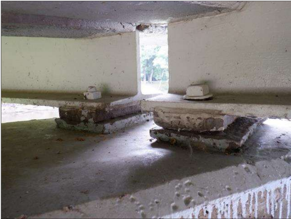
BEAM 4 BENT 1 BEARINGS
