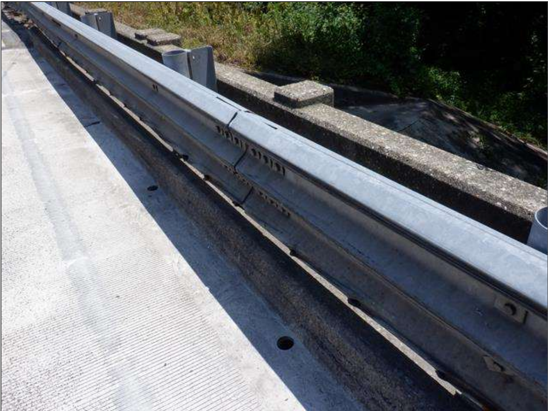
RIGHT BRIDGE RAIL
