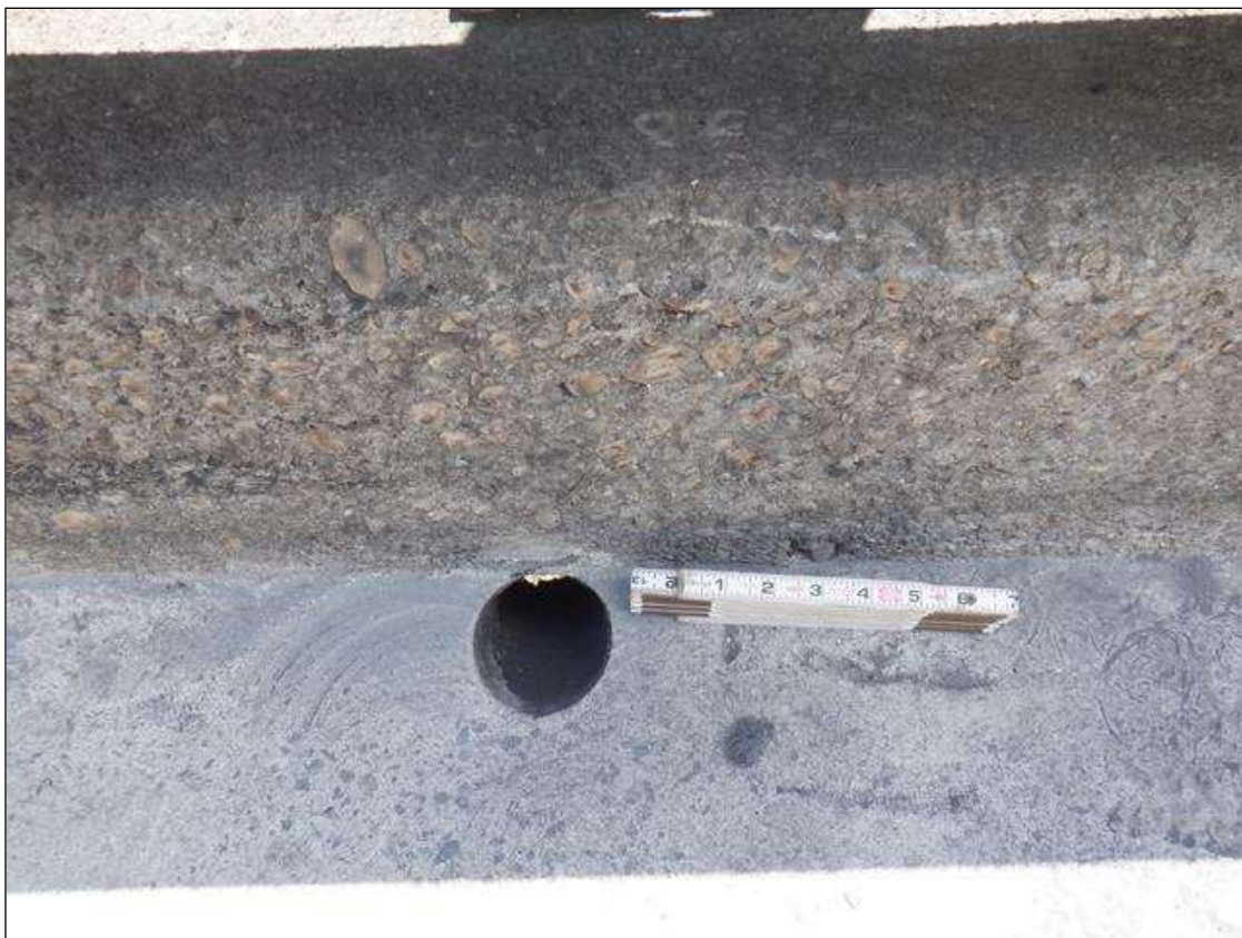
SPAN 8 ALONG RIGHT BRIDGE RAIL 3 INCHES DIAMETER SCUPPER
