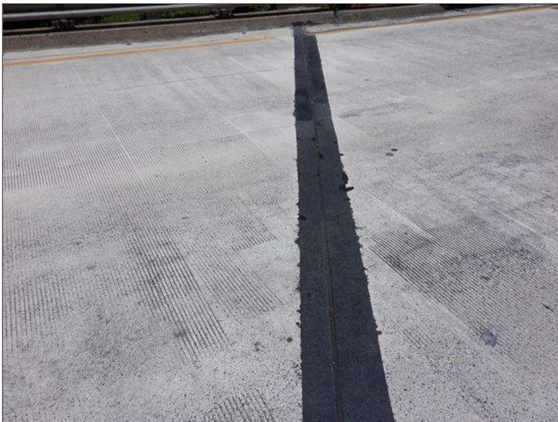
END BENT 2 JOINT
