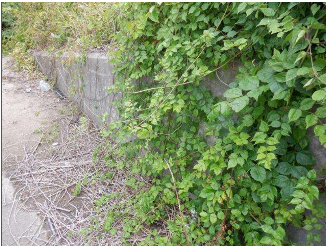
SOUTHEAST CORNER WINGWALL
