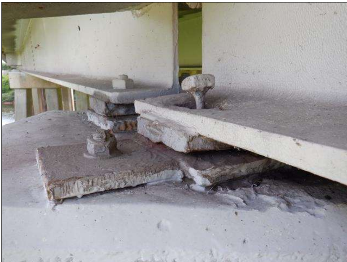
Span 1 Beam 1 - Far Bearing: WELDED REPAIR, WITH ADDED ANCHOR BOLT.
